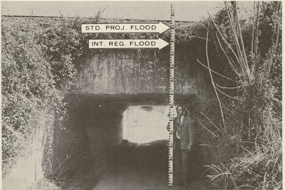
Sunset Avenue Bridge (Va. Route 781)
