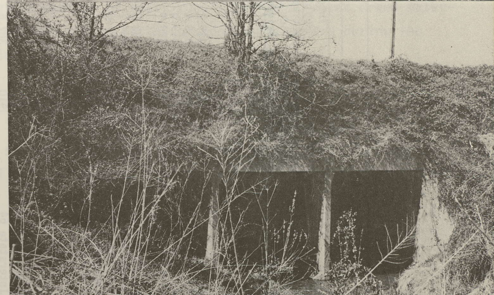
Figure 5 BRIDGES ACROSS MOORES CREEK
