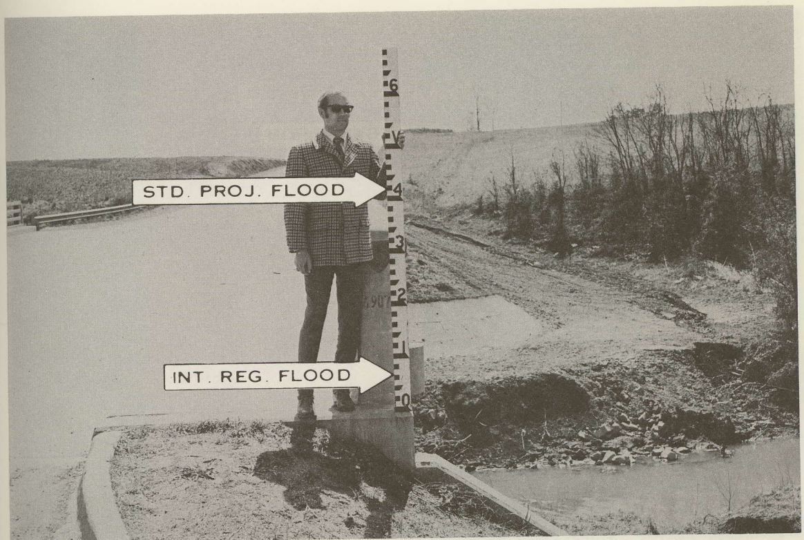
Avon Street Bridge (Va. Route 742)
