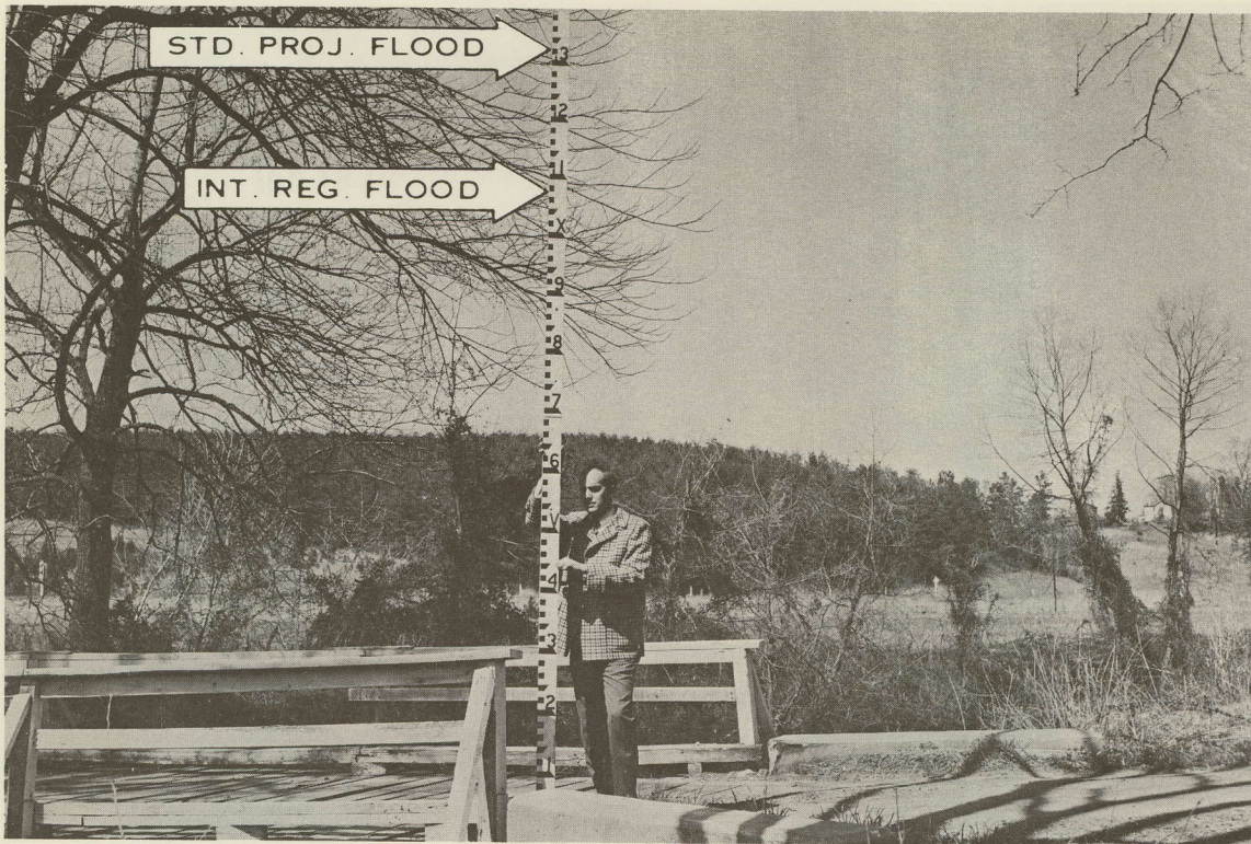
Bridge over Biscuit Run just upstream from its confluence with Moores Creek. (O'Neill Enterprises)
