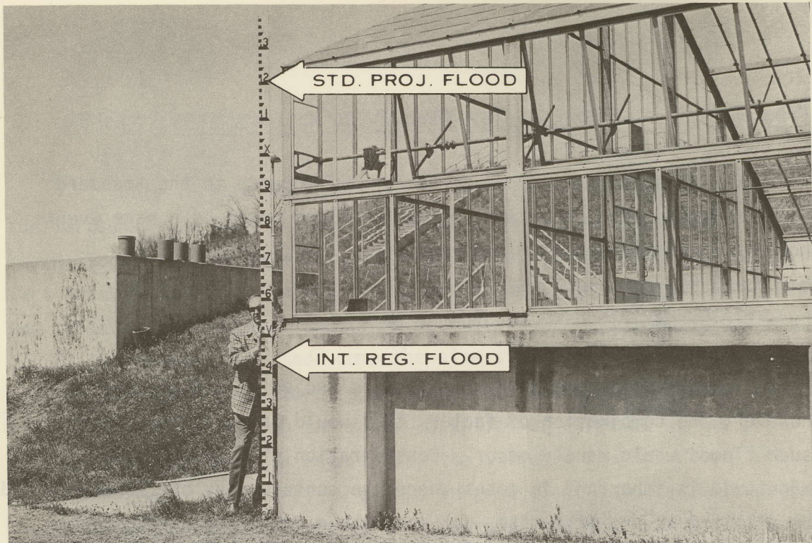
Sewage Disposal Plant
