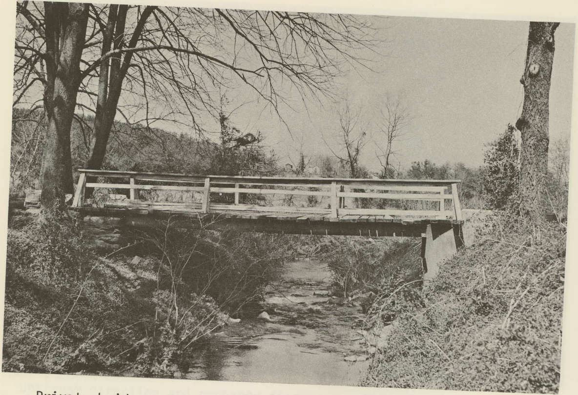
Private bridge near mouth of Biscuit Run, (O'Neill Enterprises) "WILLOWBY" DRIVEWAY BRIDGE BUILT BY COL. U.S. GRANT FOR COL. L.J. OWEN IN 1932 (GRANDSON OF GEN. GRANT)
